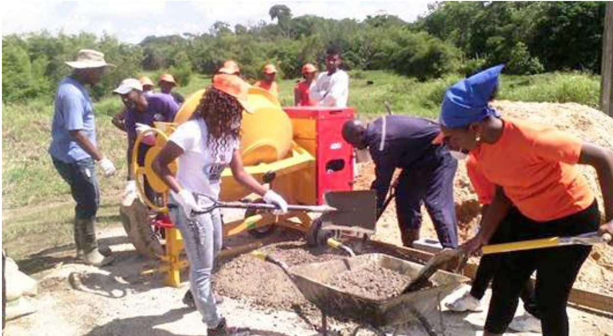
Figure 7 Trainees assisting with the mixing of concrete
